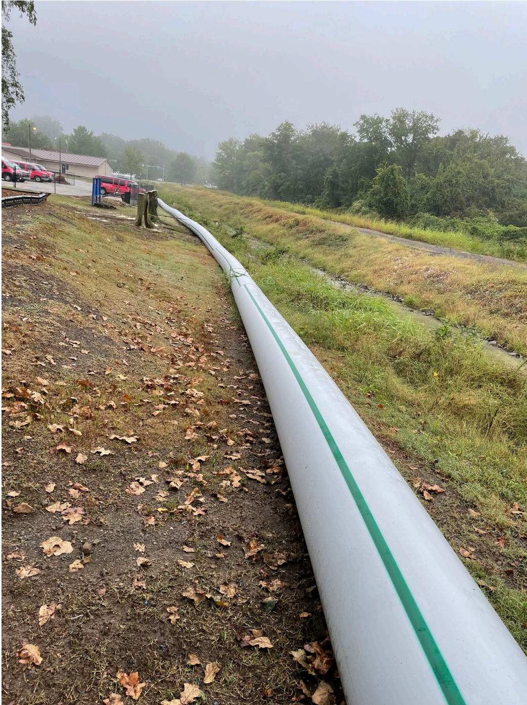
Welded HDPE Pipe Waiting To Be Installed
